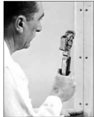
Joints are reinforced with Kal-Mesh fiberglass webbing. Steel corner and casing beads protect corners.
