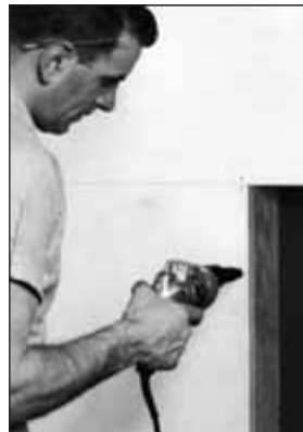
SCREW APPLICATION Fast, positive, fewer heads to treat.
