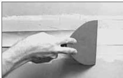
1. Fill Joint And Bed Tape Simultaneously
