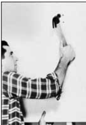
DOUBLE NAILING Minimizes nail-pop.
