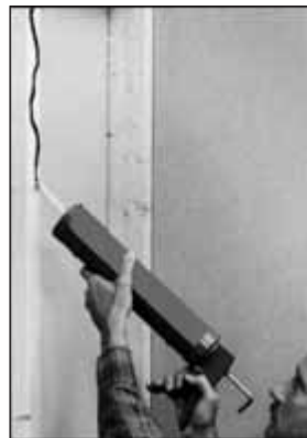
ADHESIVE/NAIL-ON Ideal for prefinished boards.
