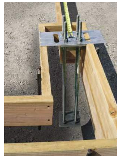
Strong Frame OMFSL anchorage assemblies make design and installation faster and easier
